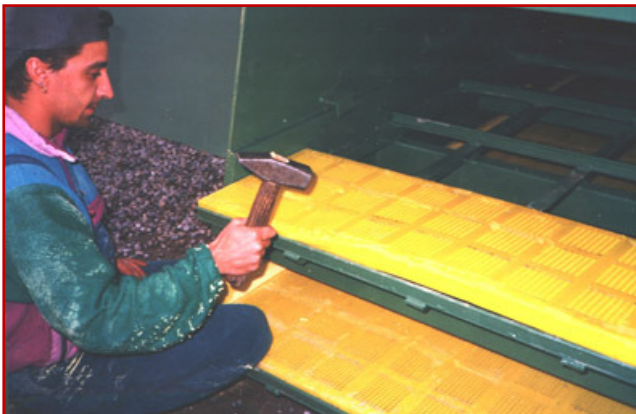
4. Press the panel with an hammer
